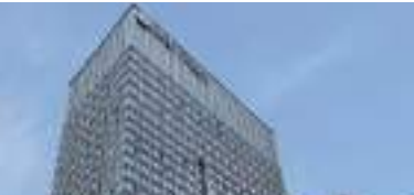
Chengdu Poly Metropolis
